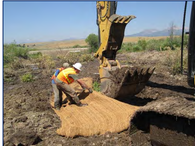
Crews install a bioengineered streambank in Reach 1
