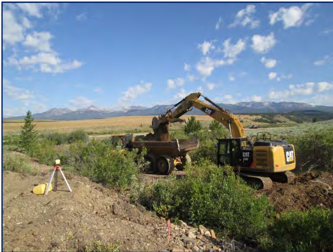
Placer tailings being removed from Reach 1. Laser (left) and excavator (right) show height of placer piles removed from Reach 1 floodplain
