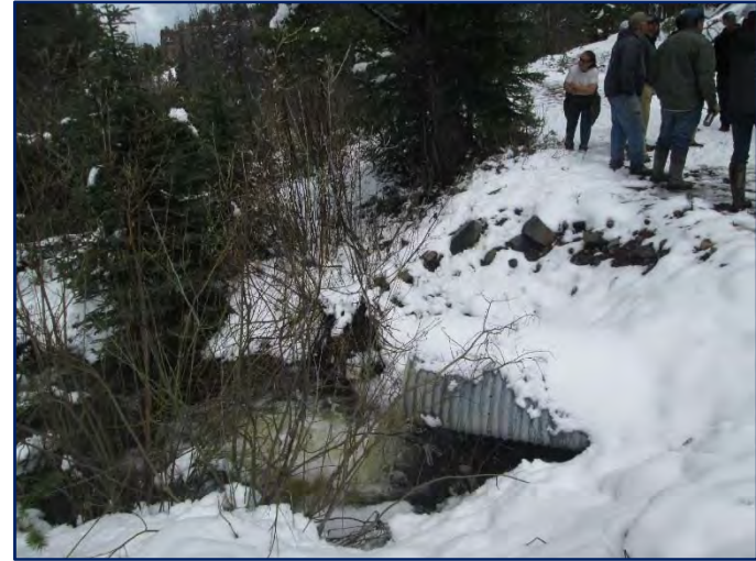
Perched culvert at the top of reach 5 shown in 2014 (left) and during pre-construction walk-through in the spring of 2016 (right)
