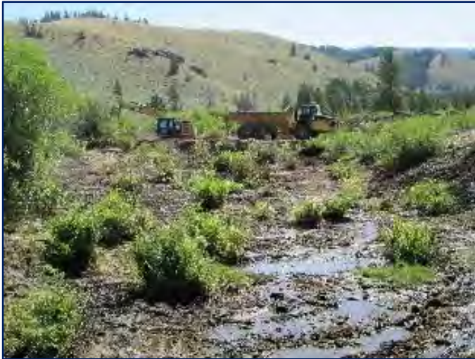
Construction equipment clearing placer piles in Reach 1. Newly created floodplain and mechanically transplanted willows in foreground
