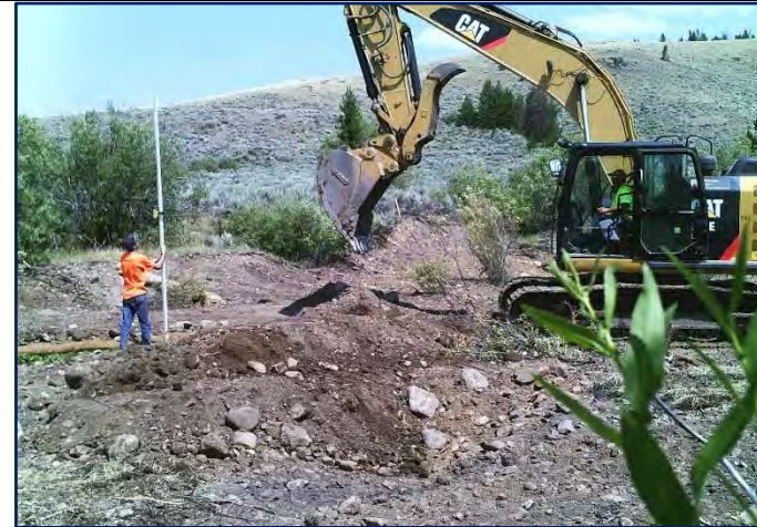
Contractors measure new streambed elevation during construction in Reach 1
