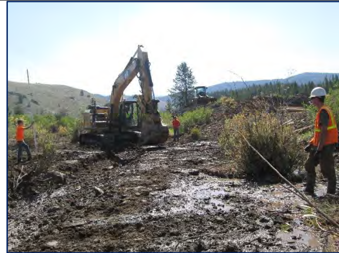
Reach 1 channel construction, showing drier floodplain areas higher in the reach (left) and where groundwater was captured (right).
