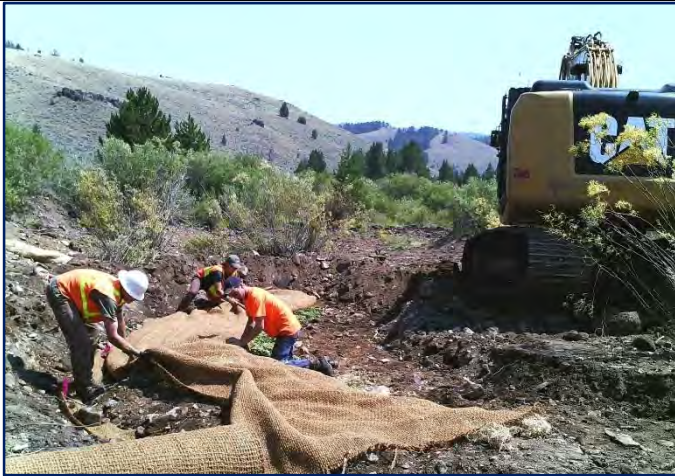
Bioengineered streambank installation in Reach 1
