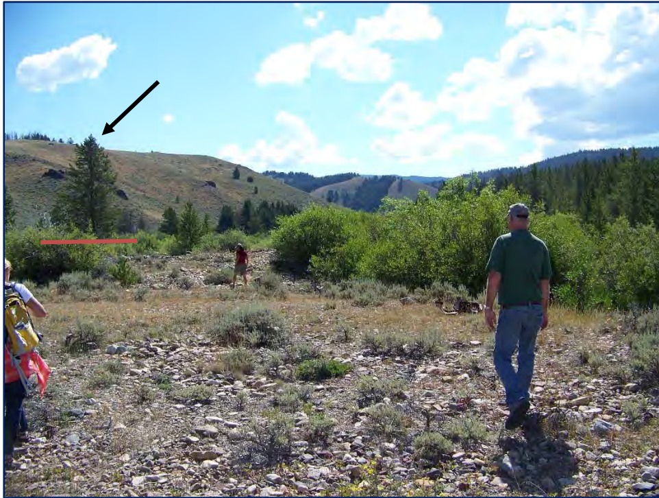
Pre-construction conditions in Reach 1, July, 2015 – tree and red line show ground level at top of placer tailings before construction
