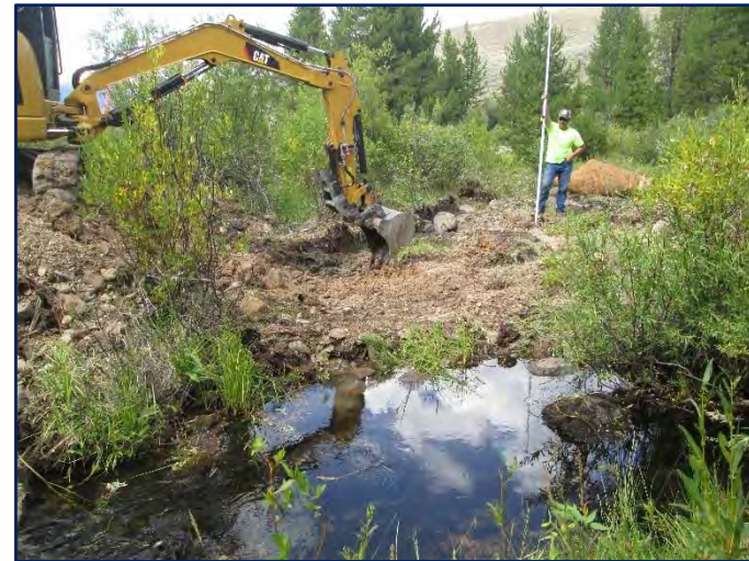
Channel construction at the top of Reach 1 (left) where new channel was tied into existing stream (right).
