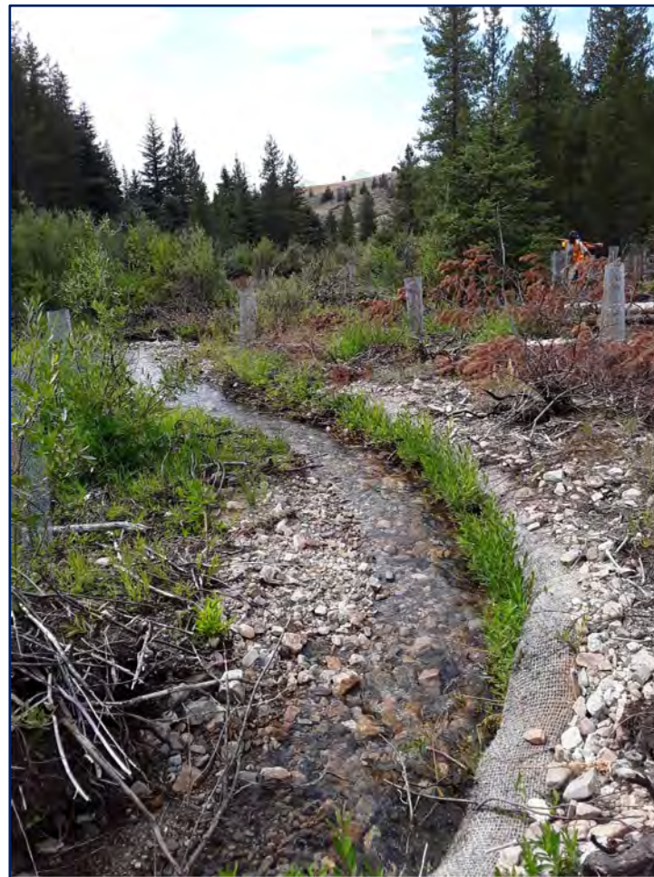
Good survival of willow whips on constructed banks from this August, 2017 image in Reach 5
