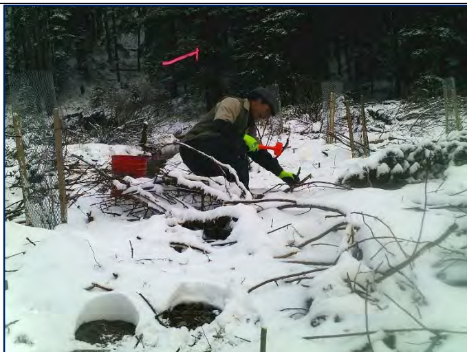
Contractors install willow stakes along riparian area of new channel- October, 2016
