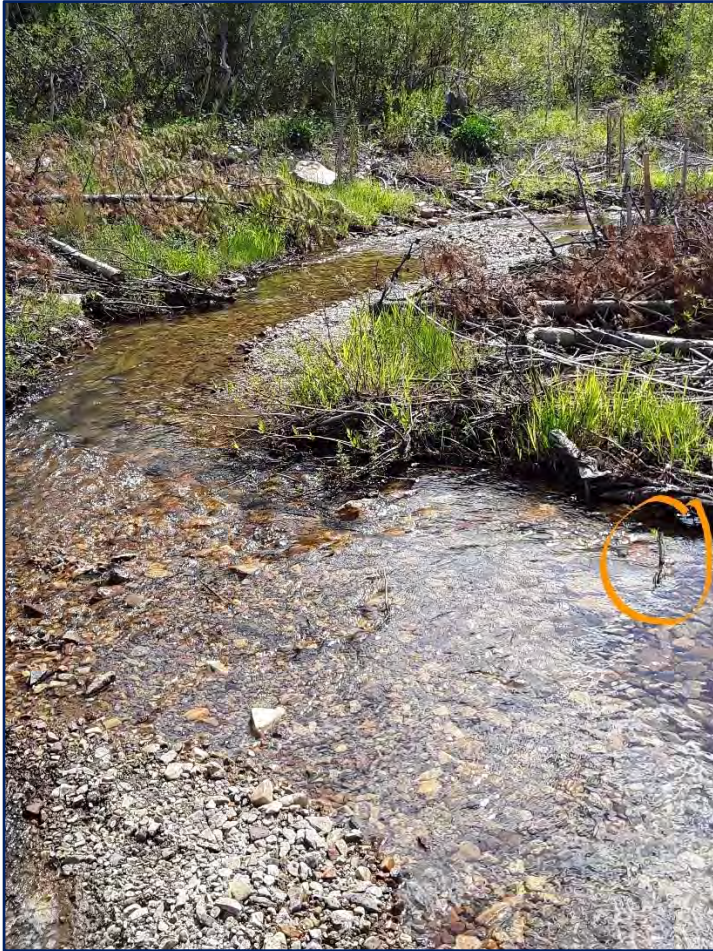
Reach 3 constructed channel section shown in August, 2017 photo. Willow stake in the circle had been planted on a bank, demonstrating channel deformity occurring, as planned
