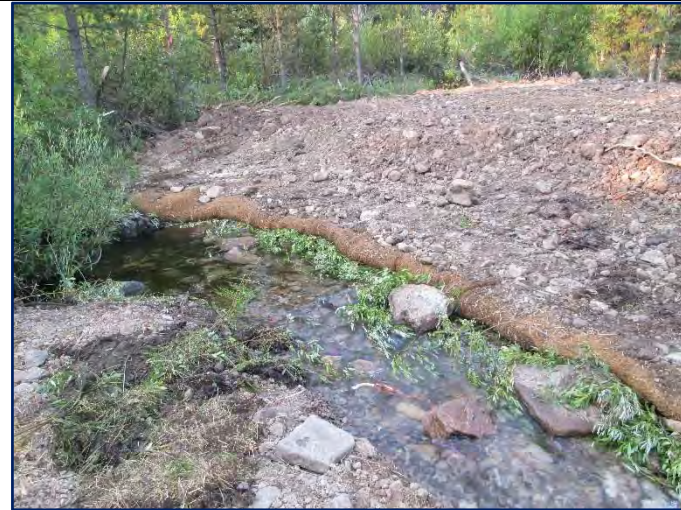
Same location where new channel was tied into existing stream. Earthen plug installed to prevent stream from returning to old channel
