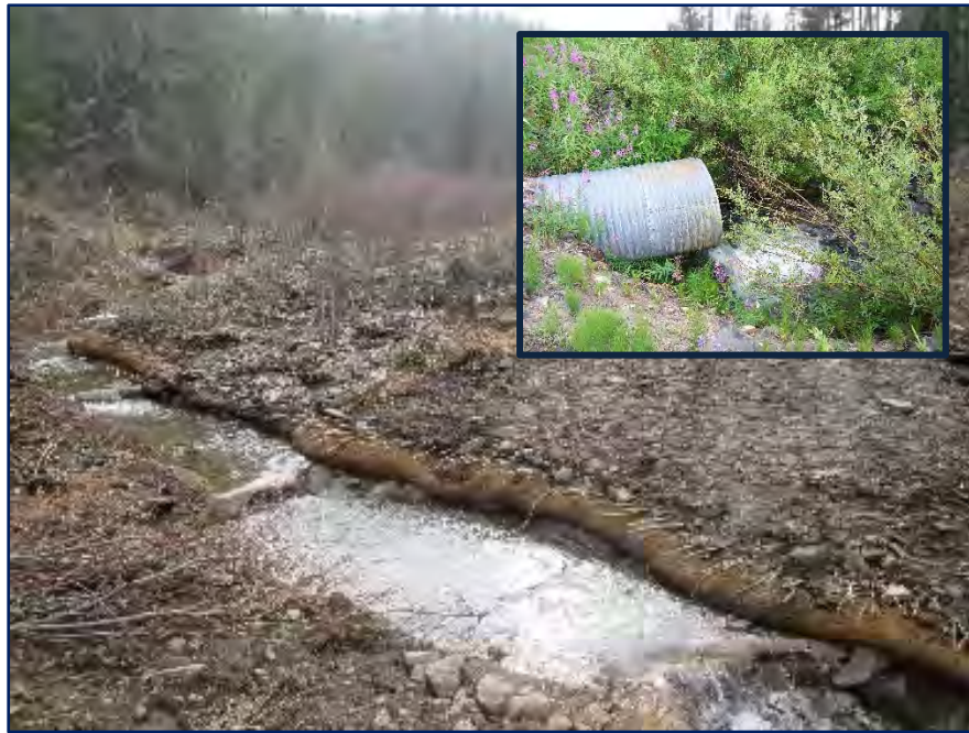
FIGURE 20. STEP-POOL FEATURE AT TOP OF PROJECT AFTER CULVERT REMOVAL (INSET IMAGE OF CULVERT FROM 2014)
