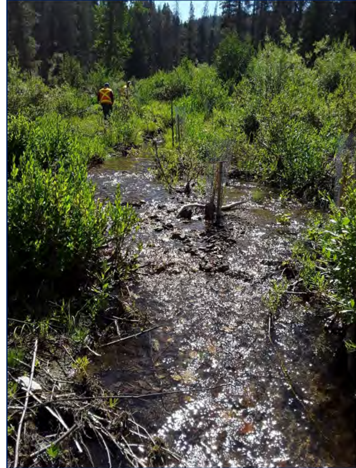
Reach 5 constructed channel showing stream movement onto the floodplain in August, 2017 image. Netted plants denote location of constructed bank in 2016
