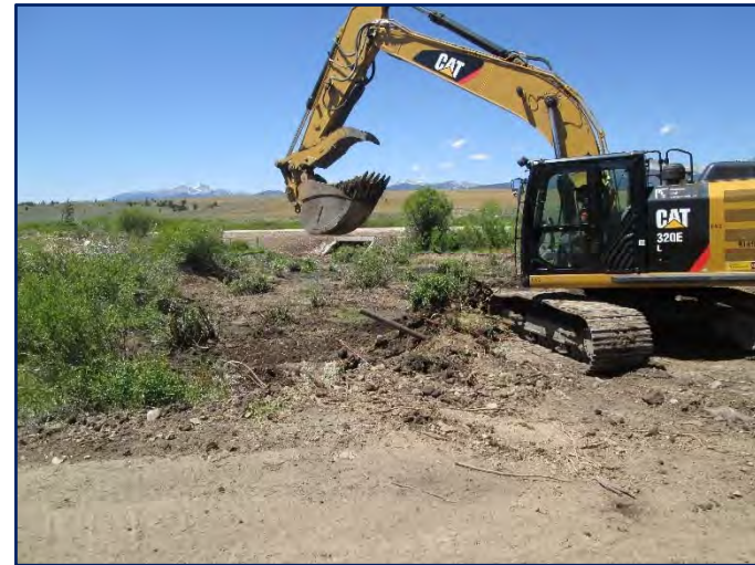
Placer tailings being removed from Reach 1. Laser (left) and excavator (right) show height of placer piles removed from Reach 1 floodplain
