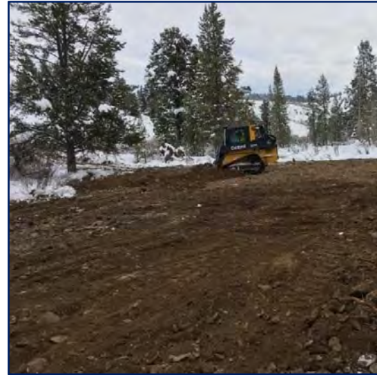
Overbank flows accessed staging/parking area in Reach 2 in May, 2017 (left) prompting additional work to be implemented in November, 2017 to add over 2 feet of material to the floodplain (right)
