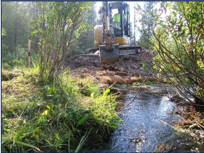
Building a bioengineered bank at the top of Reach 1.
