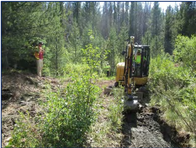
Channel construction at the top of Reach 1 (left) where new channel was tied into existing stream (right).
