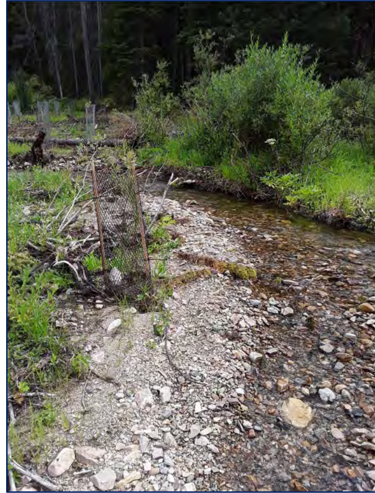
Point bar formation in mid-August, 2017 on constructed channel in Reach 2
