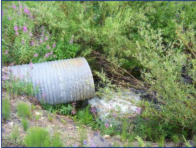
Perched culvert at the top of reach 5 shown in 2014 (left) and during pre-construction walk-through in the spring of 2016 (right)
