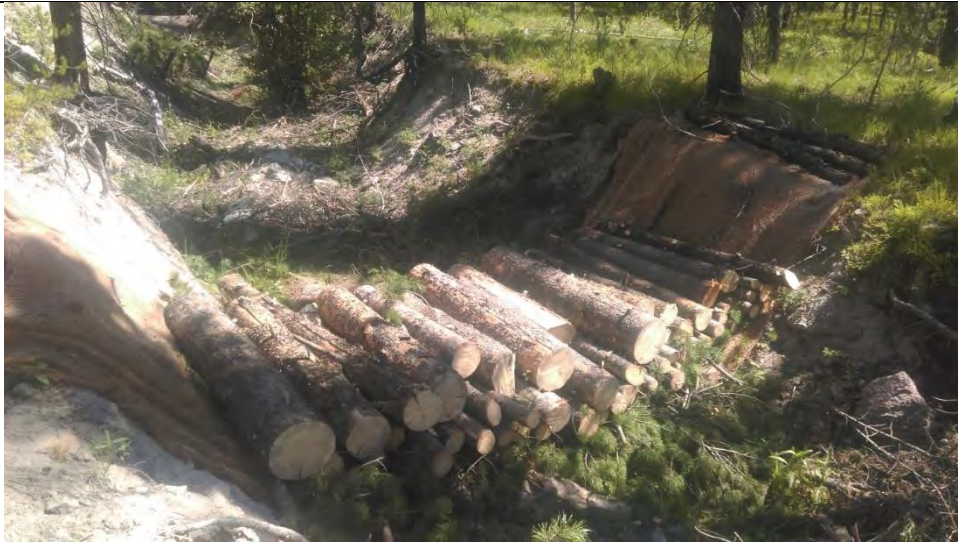
Example of enhanced SSR-2d structure previously filled (above) and SSR-2c slash filters in gully bottom and bank walls (below)
