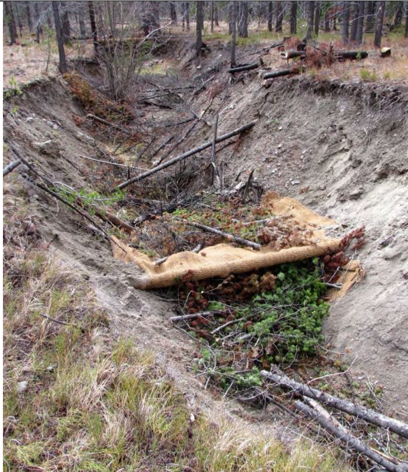
Coir-lined fabric in gully above California Creek taken in Fall 2015 (left) and Spring 2016 (right). This gully captured overland flow and gully structures below held back water and promoted vegetation establishment previously non-existent. Bank slope lengths also reduced from slash filters.
