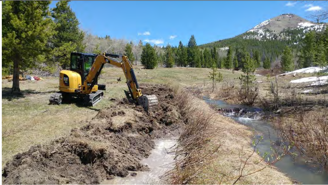
Installation of willow brush trench in California Creek. Disturbed soil was seeded and capped with brush to minimize soil loss (October 2016)
