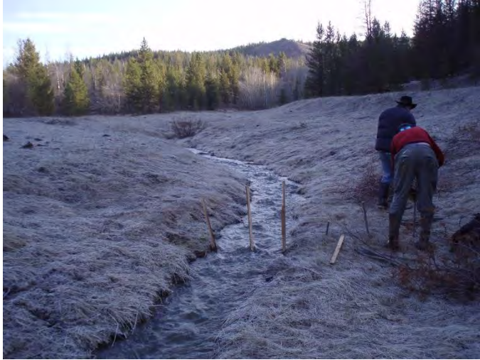
Figure 27. SSR-2b (Beaver Mimicry structures) examples
