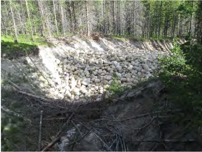
Engineered rock structures installed by NRDP in two gullies above California Creek. Images (top row) looking upstream at structures from below and looking upstream at structures from above (bottom row)
