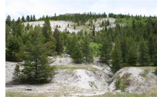
Image 1: Bare areas and Gullies drain under highway to Mill Creek
