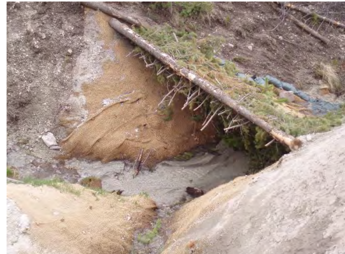
SSR-2d structure before (top) during (bottom left) and immediately after installation in 2014 and one year later with some sediment catchment (bottom right)
