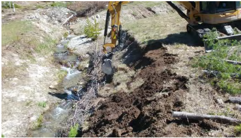
Example of brush bundle installation and mechanical enhancement in California Creek: Summer 2013 (top left); Spring 2015 (top right); Spring 2017 (bottom and next page)
