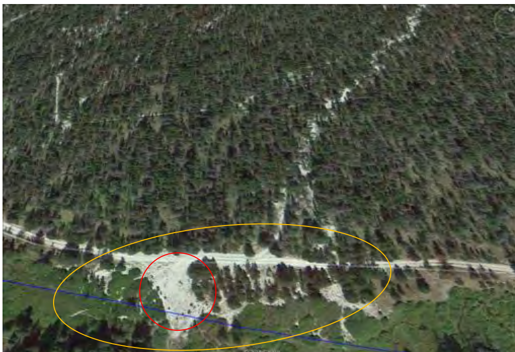
Figure 13. Sediment plume and gully above California creek. The more active plume area shown in the red circle and the historic plume shown in the orange and the contributing gullies were treated by NRDP and DEQ in 2014.
