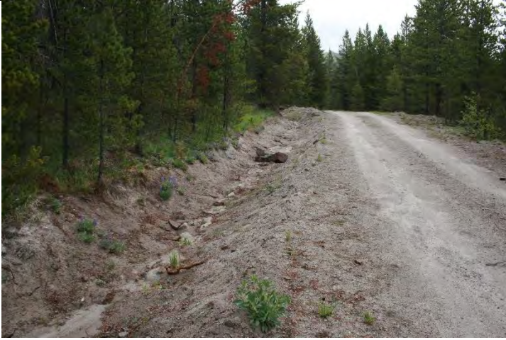
Road work area (above) with improved roadside drainage and expanded catchment area at base. Culvert remains plugged and will be addressed by MFWP in the future. Culvert removal from stream in California Creek shown below and on next page
