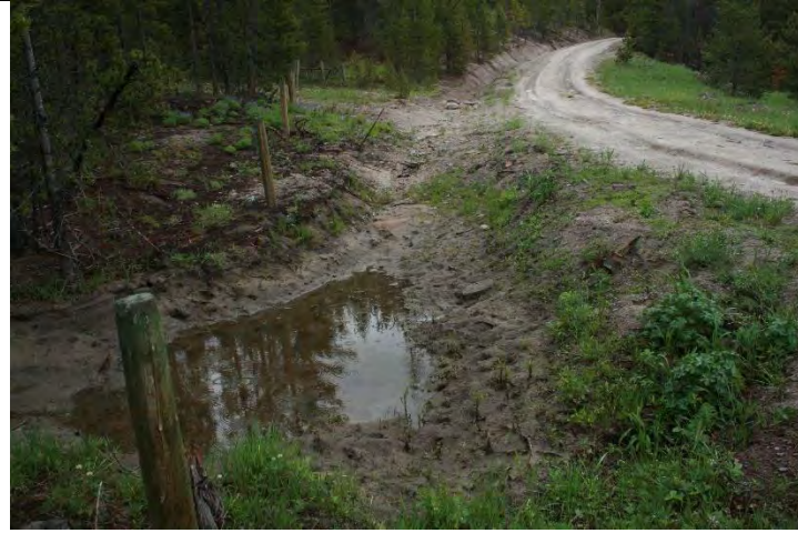
Road work area (above) with improved roadside drainage and expanded catchment area at base. Culvert remains plugged and will be addressed by MFWP in the future. Culvert removal from stream in California Creek shown below and on next page
