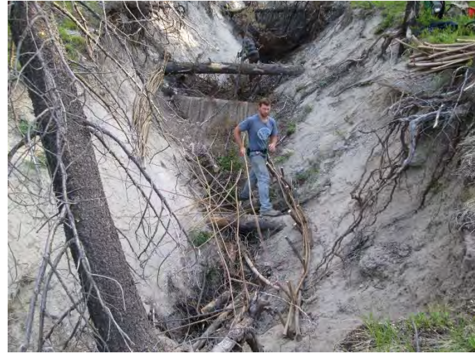
Example of gully structures. Some filled structures were re-visited in 2016 and gullies were brought up to grade (bottom right).
