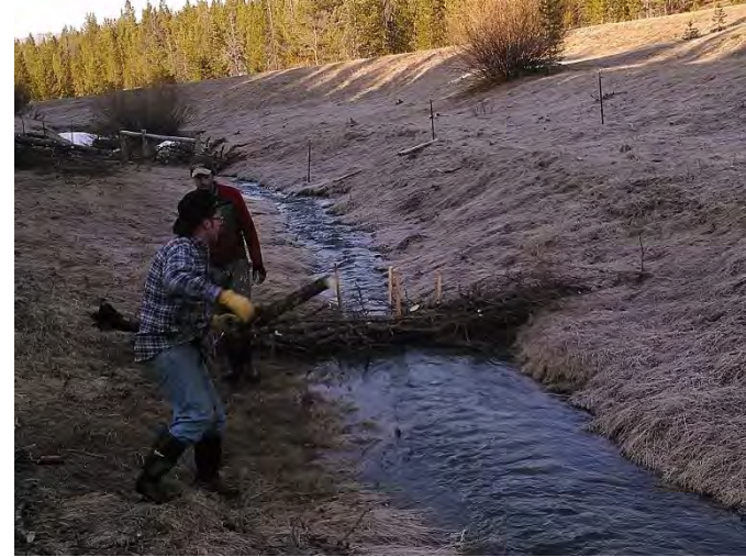
Figure 27. SSR-2b (Beaver Mimicry structures) examples
