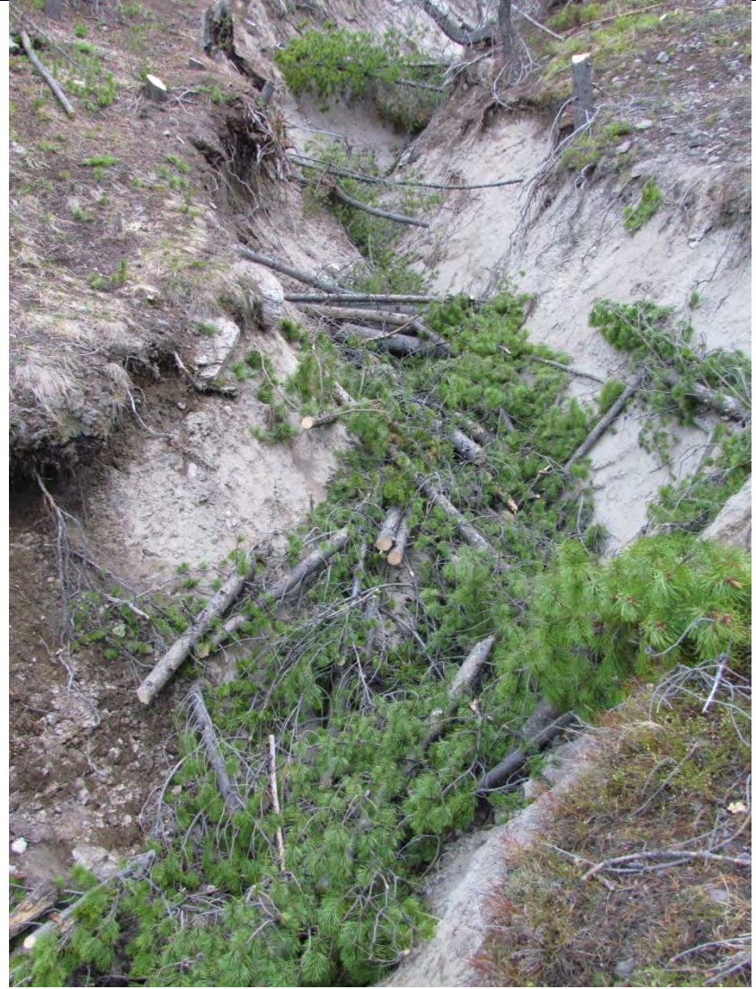
Gully slash filters in gullies above California Creek soon after installation in 2014
