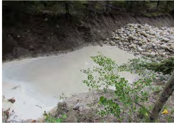
Rock check dams filled with sediment and runoff in California creek drainage.
