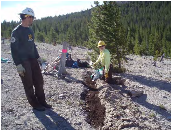
Compost soil amendment in trench
