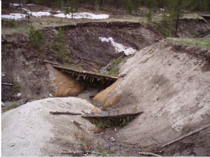
Mechanized enhancement to eroding banks in 2017, including deposition of erosion into existing structures
