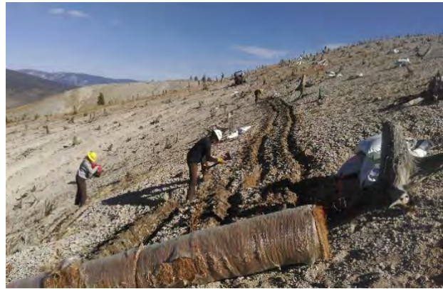
Seeded and fertilized micro-swales (trenches) are installed before being covered by coconut coir erosion fabric and fastened with stakes and woody debris in Joyner Gulch
