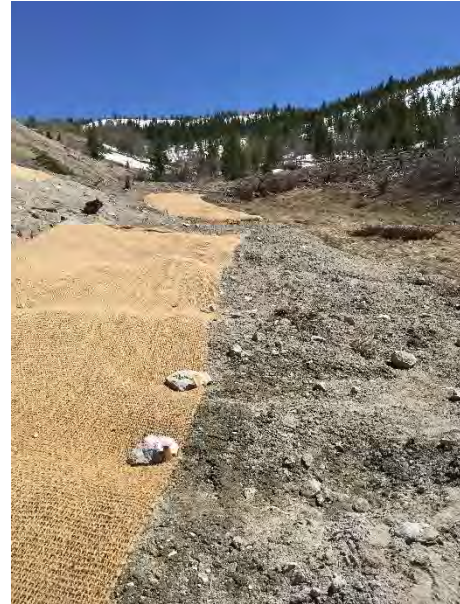
Filled gully matches existing slope angle. Stream here was redirected to old channel through sedge mat at new low point in valley
