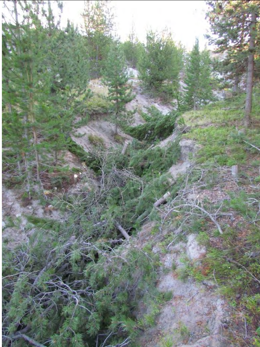
Gully slash filters in gullies above California Creek soon after installation in 2014
