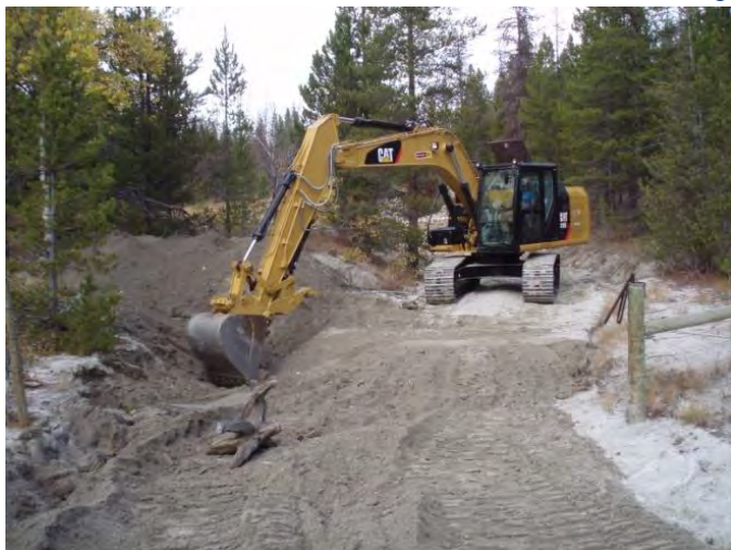
Digging catchment beside plume area (top left) and view across road where large rill used to cross (top right) in California Creek. Road work area 3 (below) right showing ditch and culvert crossing
