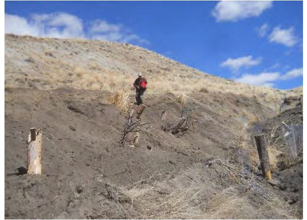
Broadcast seeding via hand-operated belly seeder on freshly worked soil adjacent to a gully.
