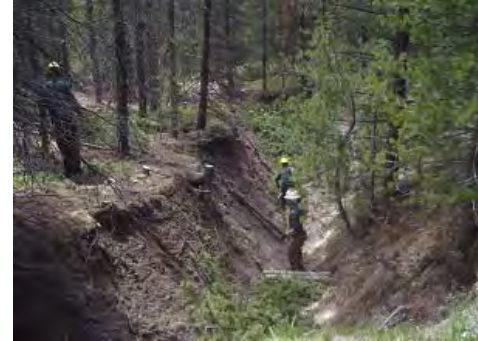
Image 1. C.31 Steep gullie slopes being stabilized with SSR-2d structures
