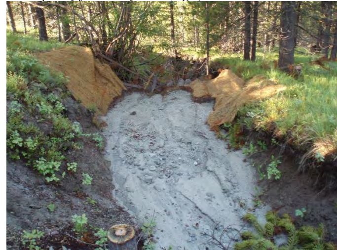
Gully structures using coir fabric after 1 year of sediment delivery in upper California Creek
