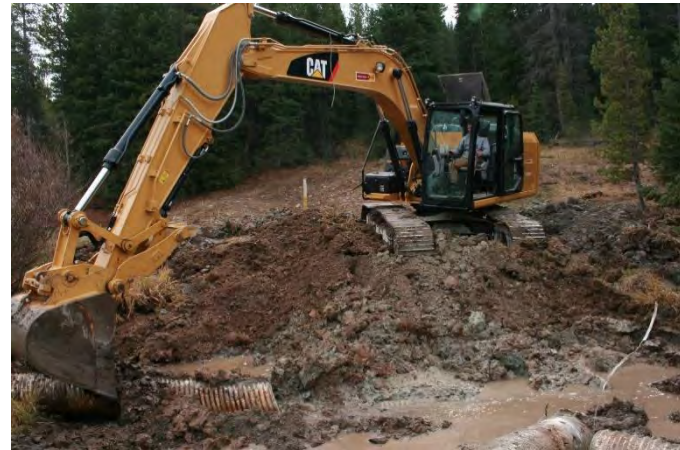
Road work area (above) with improved roadside drainage and expanded catchment area at base. Culvert remains plugged and will be addressed by MFWP in the future. Culvert removal from stream in California Creek shown below and on next page
