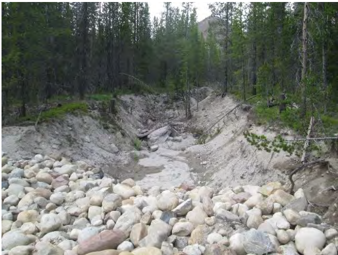
Engineered rock structures installed by NRDP in two gullies above California Creek. Images (top row) looking upstream at structures from below and looking upstream at structures from above (bottom row)
