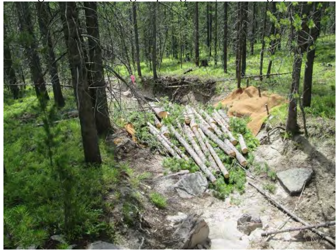
Example of gully structures. Some filled structures were re-visited in 2016 and gullies were brought up to grade (bottom right).
