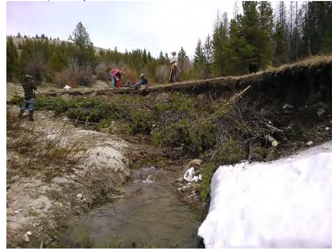
Example of brush bundle installation and mechanical enhancement in California Creek: Summer 2013 (top left); Spring 2015 (top right); Spring 2017 (bottom and next page)
