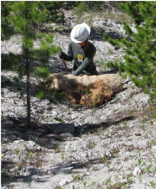
Rill treatment structures installed by MCC crews, June 2014
