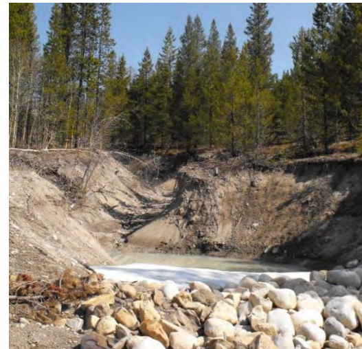
Engineered rock structures installed by NRDP in two gullies above California Creek. Images (top row) looking upstream at structures from below and looking upstream at structures from above (bottom row)
