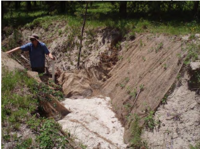
Gully structures using coir fabric after 1 year of sediment delivery in upper California Creek
