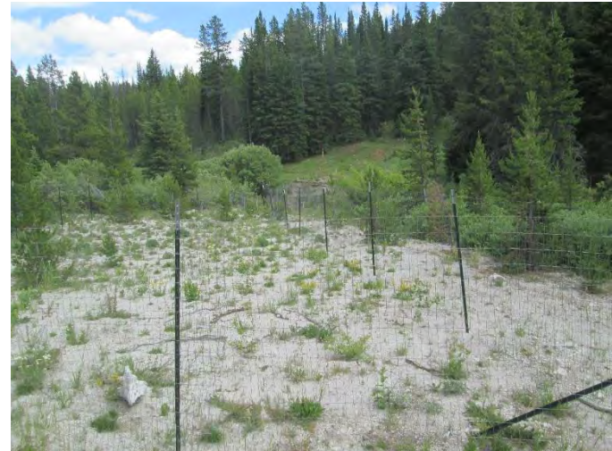
May, 2014, snowmelt from gully crosses California Creek road and adds to sediment plume (left); June, 2016 beginning of vegetation establishment after installation of culvert gully plugs and container plants (right)
