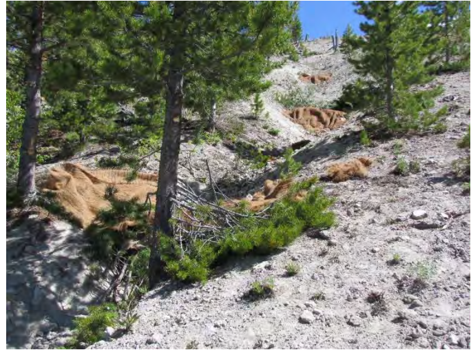
Rill treatment structures installed by MCC crews, June 2014
