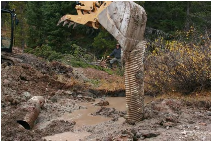
Road work area (above) with improved roadside drainage and expanded catchment area at base. Culvert remains plugged and will be addressed by MFWP in the future. Culvert removal from stream in California Creek shown below and on next page
