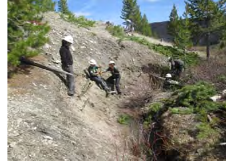
Image 2: Crews treating gully at bottom of unit in 2015
