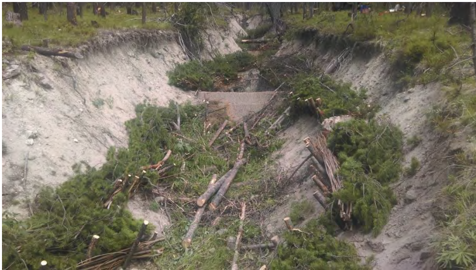
Example of enhanced SSR-2d structure previously filled (above) and SSR-2c slash filters in gully bottom and bank walls (below)
