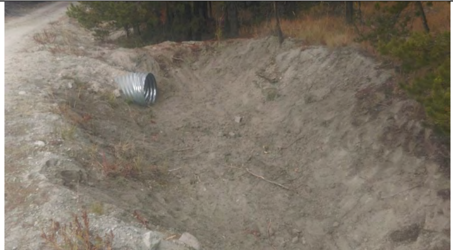
Road work area in California Creek (above) showing ditch and catchment basin. Another road work area (below) with sediment deposition from 2015 (left) and 2016 (right) spring flows
