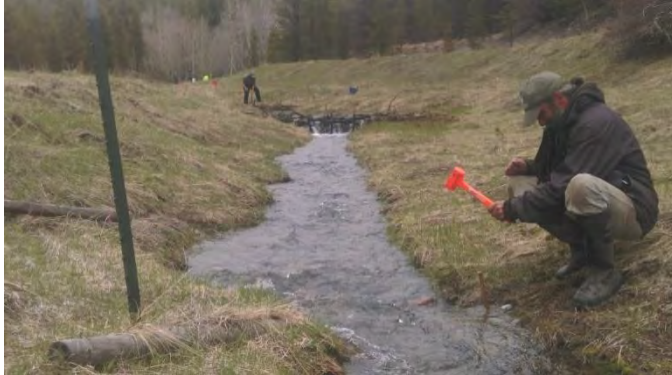
Installing willow stakes below beaver analog structure in May 2016 (above) and in June 2015 (right) in California Creek
