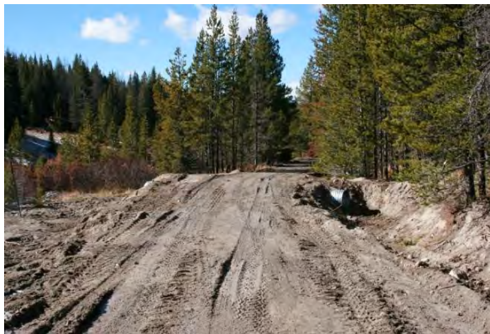
Digging catchment beside plume area (top left) and view across road where large rill used to cross (top right) in California Creek. Road work area 3 (below) right showing ditch and culvert crossing
