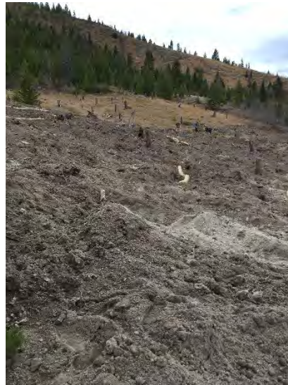
Several acres of slope pitting and roughening adds microtopography which improves water retention, planting success, and soil stability; Stucky Ridge
