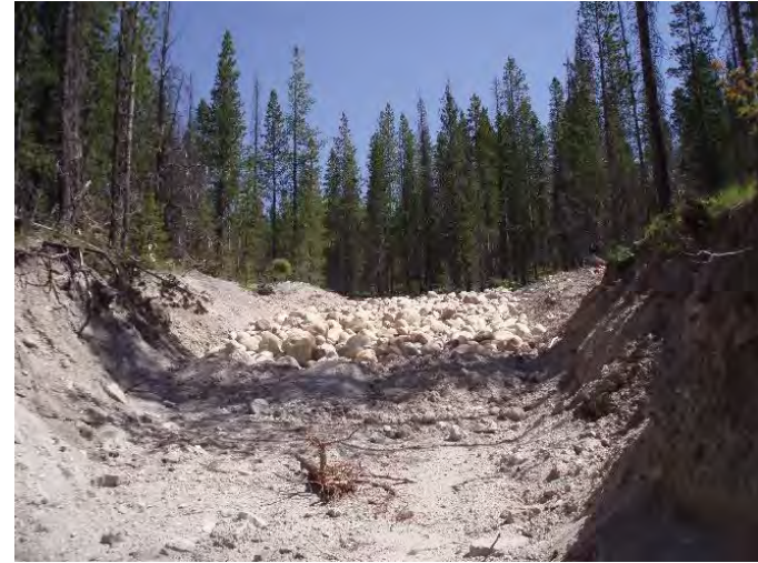
Engineered rock structures installed by NRDP in two gullies above California Creek. Images (top row) looking upstream at structures from below and looking upstream at structures from above (bottom row)
