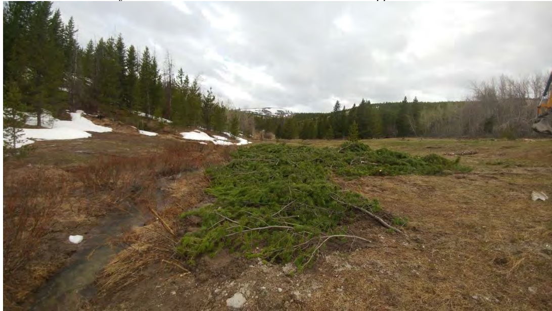
Installation of willow brush trench in California Creek. Disturbed soil was seeded and capped with brush to minimize soil loss (October 2016)
