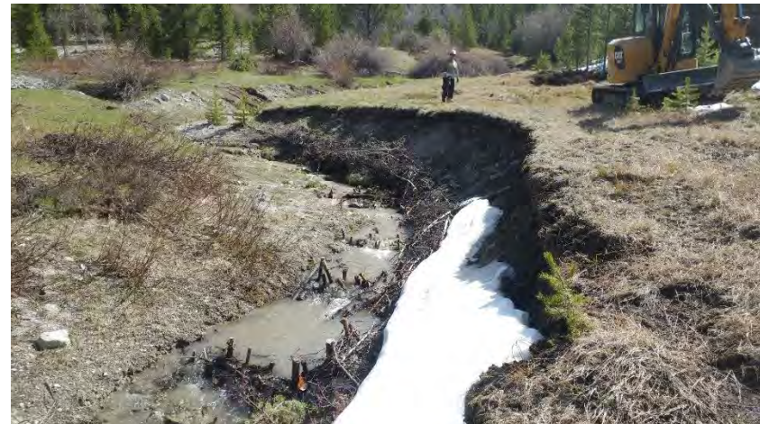
Example of brush bundle installation and mechanical enhancement in California Creek: Summer 2013 (top left); Spring 2015 (top right); Spring 2017 (bottom and next page)
