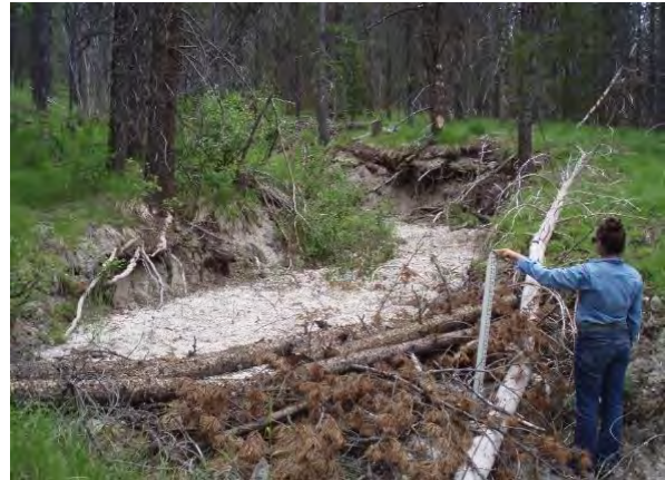
A log and slash check dam that filled with sediment over the course of one year in the Mt. Haggin WMA
