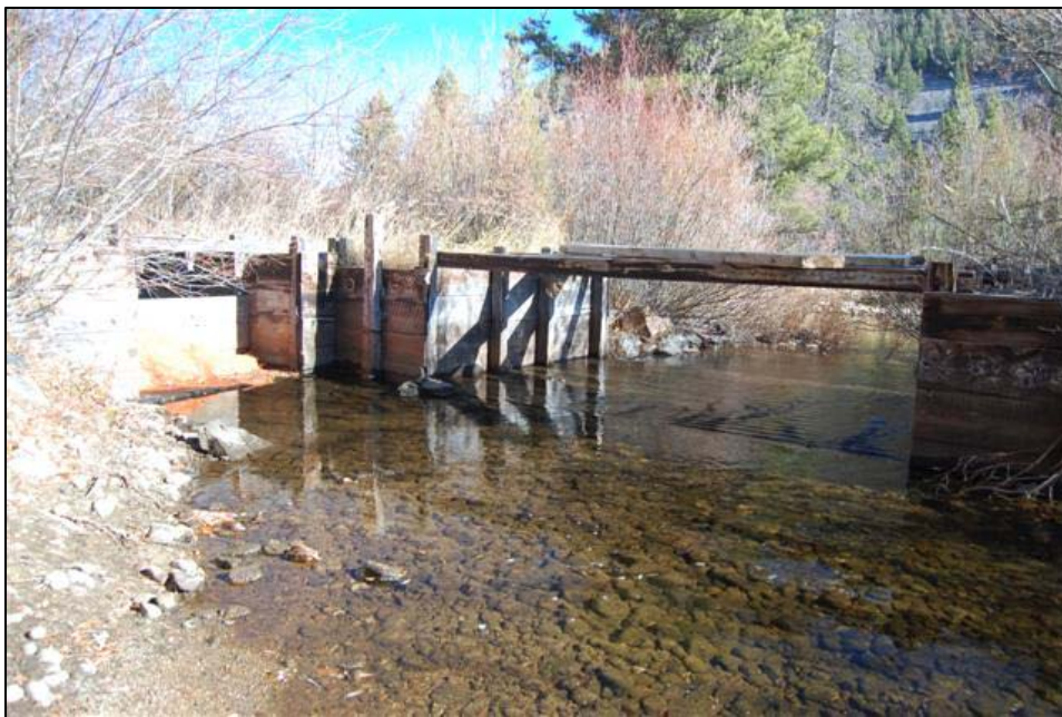
Photo 20. Split Diamond head gate and return channel at RM, 10.10, Map 6. Timber and slot board assembly.
