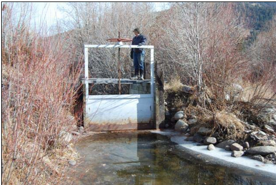
Photo 14. Truman Ditch head gate comprised of treated timber and steel gate assembly.
