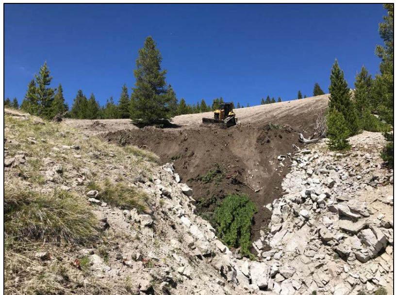
Watershed Consulting LLC filling and neutralizing an erosive gully on the Mount Haggin WMA. The machine work also consisted of roughing (dozer basins) the bare areas to give upcoming seed and fertilizer applications surface area to establish and grow.
