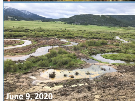
Lower French Creek, pre- and post-construction. By constructing 4,000 feet of new stream channel away from an erosive terrace, BHWC & partners removed >800 tons of sediment from the system.
