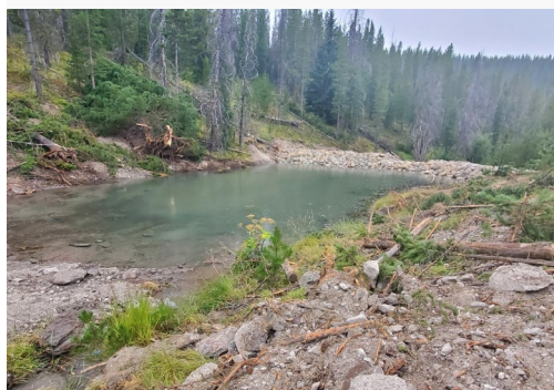
A spreader dike constructed by BHWC & partners to store water on the Mt. Haggin WMA landscape.
