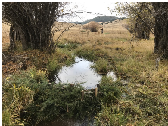
BHWC & partners have installed >120 beaver dam analogs on E. Fork Divide Creek since 2019.
