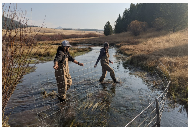
Ben LaPorte, BHWC Program Manager & Elissa Chott, Beaver Conflict Resolution Field Tech., Clark Fork Coalition, installing a beaver culvert fence at the Mule Ranch.
