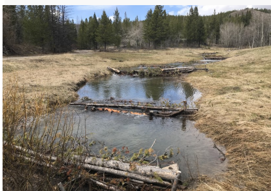
Third generation beaver mimicry structures have widened California Creek's wetted perimeter 5x.
