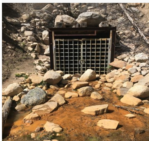
This adit, or horizontal mine shaft, at the historic Elkhorn Mine contributes bright orange, metals-laden contamination to Elkhorn Creek & the surrounding area.
