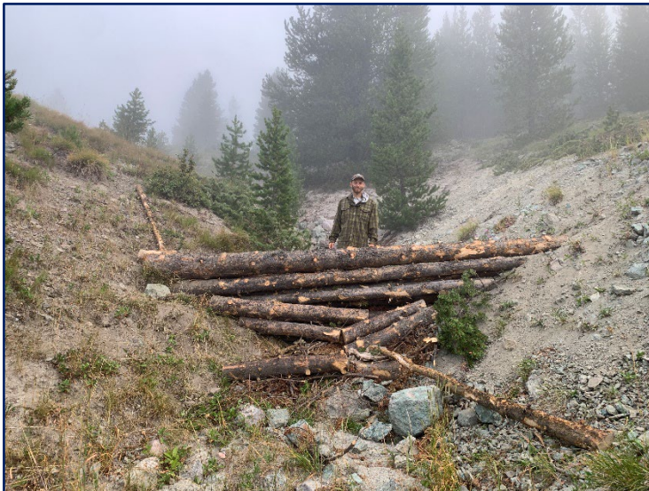
Newly constructed gully check dam (2022).
