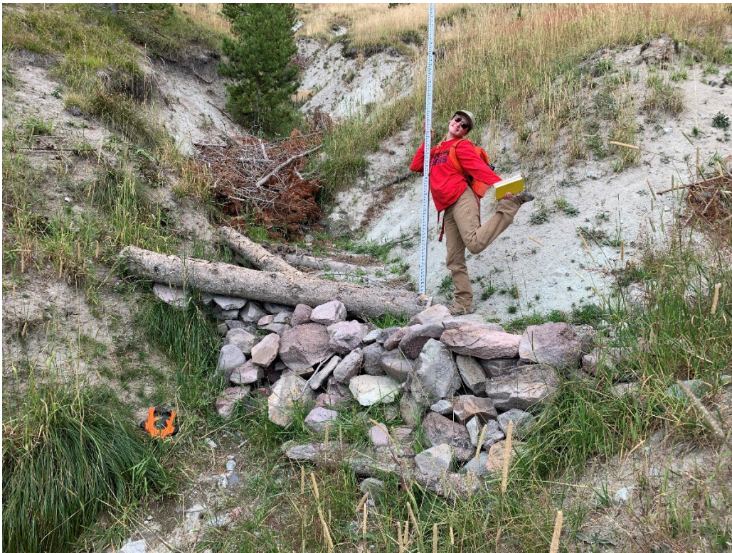
Figure 7. BHWC intern measuring captured sediment behind 3 different gully check structures
