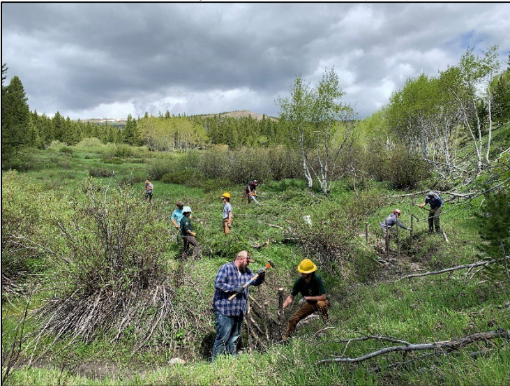
MCC and volunteers building in-stream structures in the middle reach (2022).
