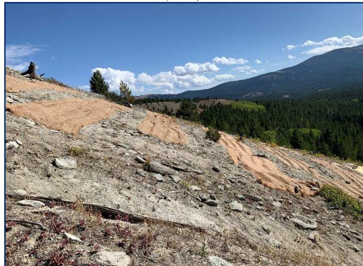
Freshly constructed "coir band-aids" in the uplands (2022).
