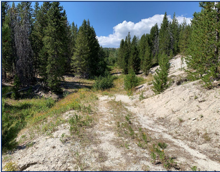
Before photo of road obliteration (2022).
