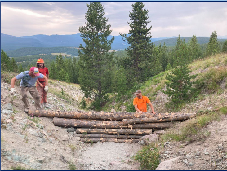
Newly constructed gully check dam (2022).
