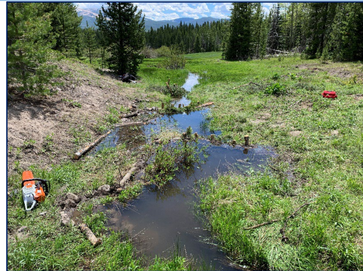
Newly constructed BDA series in the upper reach (2022).
