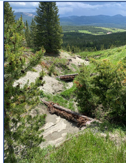
Gully check dam series holding back freshly deposited sediments (2023)
