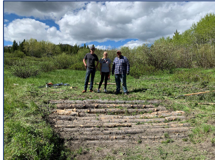
Volunteers proud of their work on a large head-cut stabilization structure in the middle reach (2022).
