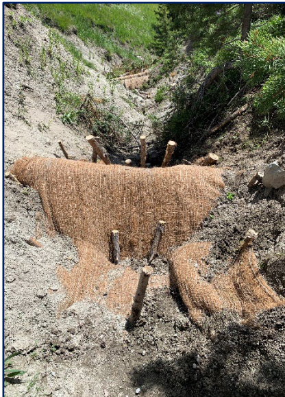
Gully check dam maintenance (2023).
