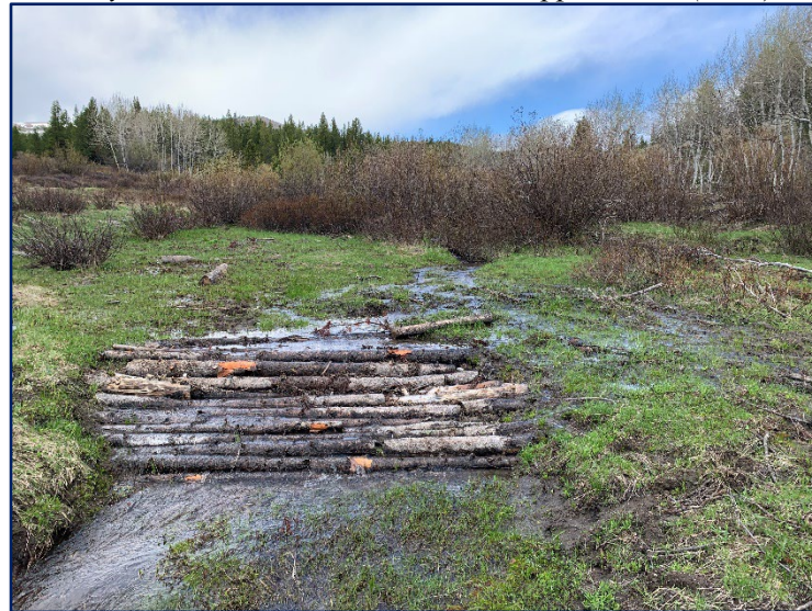
Large head cut activated and properly functioning (spring, 2023)
