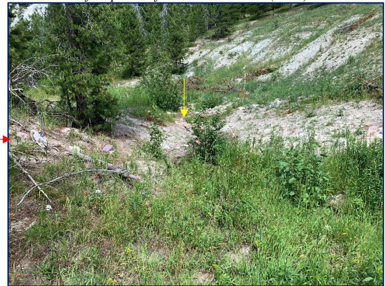
After photo of perched culvert removal (2023).
