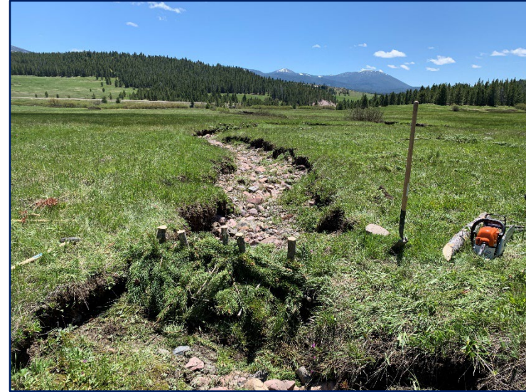
Completion of BDA in the lower reach (2022).
