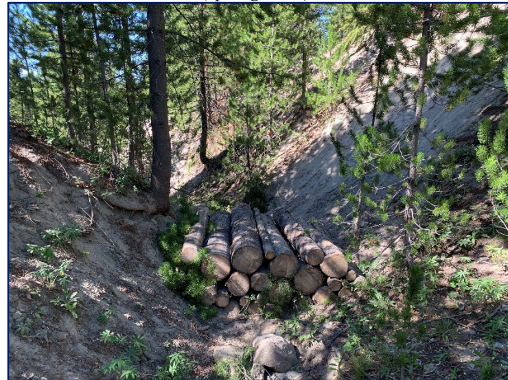
Newly constructed gully check dam (2022).
