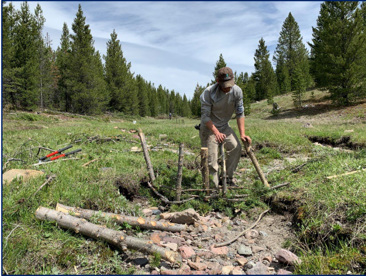
Installation of lower reach BDA (2022).
