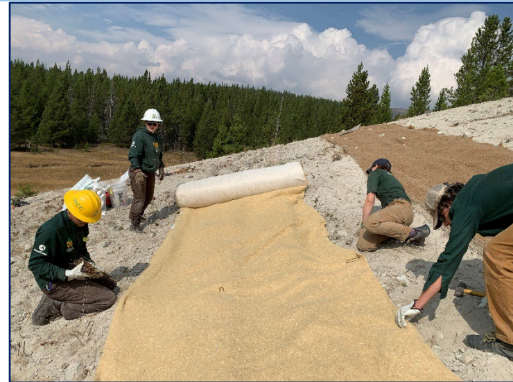
Coir being installed over trenches and fertilizer, mid construction (2022).
