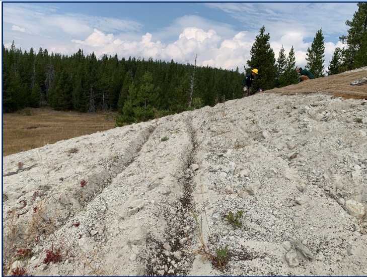
Scarification trenches and fertilizer in "coir band-aid", mid-construction (2022)
