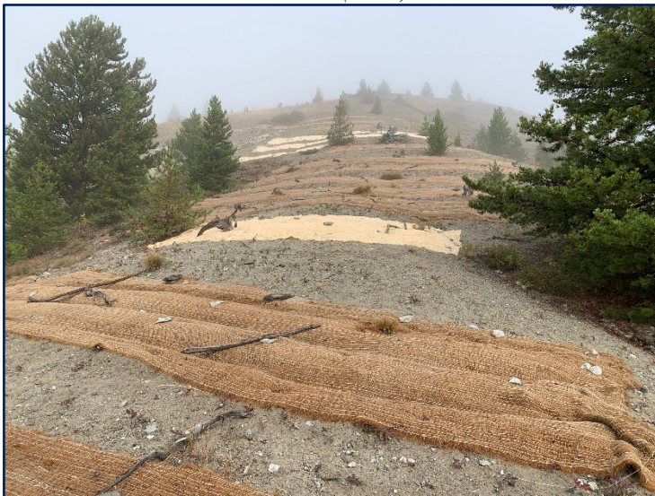
Freshly constructed "coir band-aids" in the uplands (2022).
