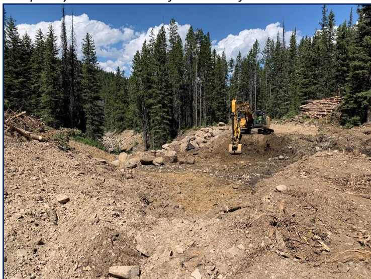
Subgrade excavation and stockpiling of boulders used for step pool construction.
