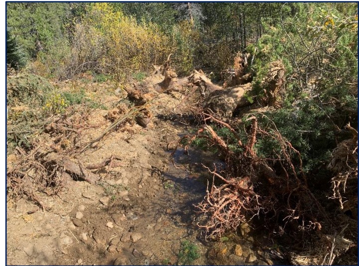
Looking downstream second eroding bank/stream crossing post-restoration. Note the large root was anchored into both sides.
