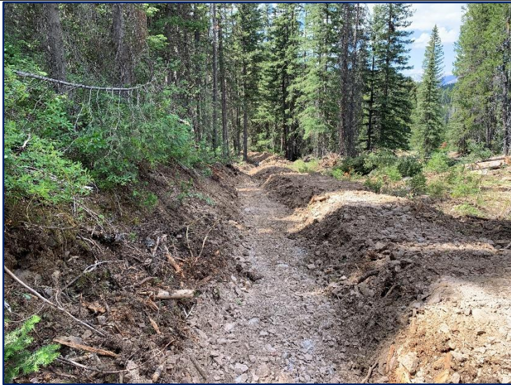
Temporary diversion ditch construction prior to plastic lining.
