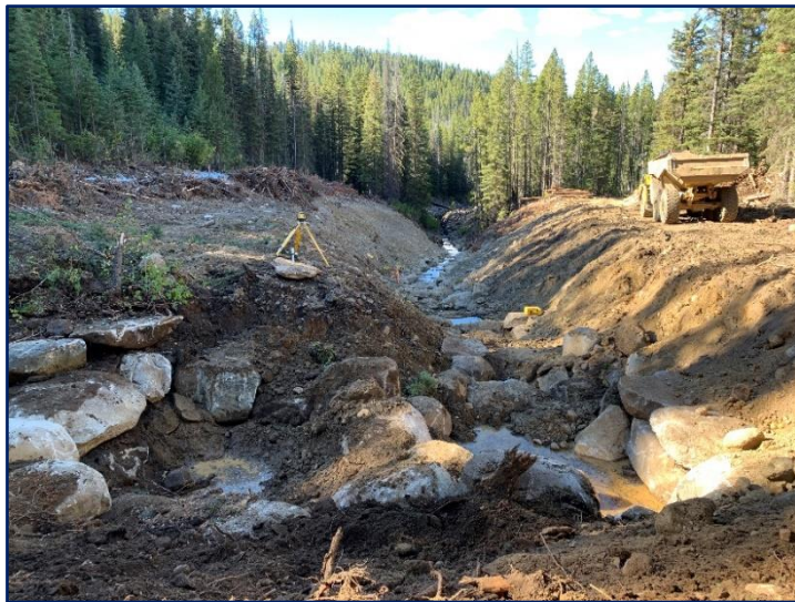
Dry step-pool structure before stream activation.
