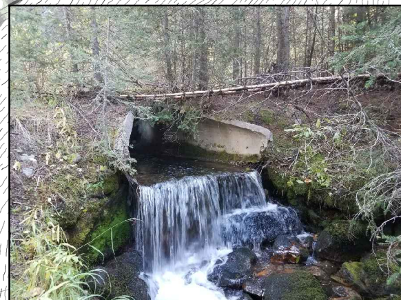
EXISTING RCP CULVERT
