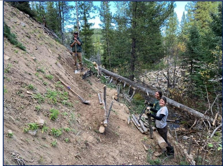
Wattle fence construction with the MCC crew.
