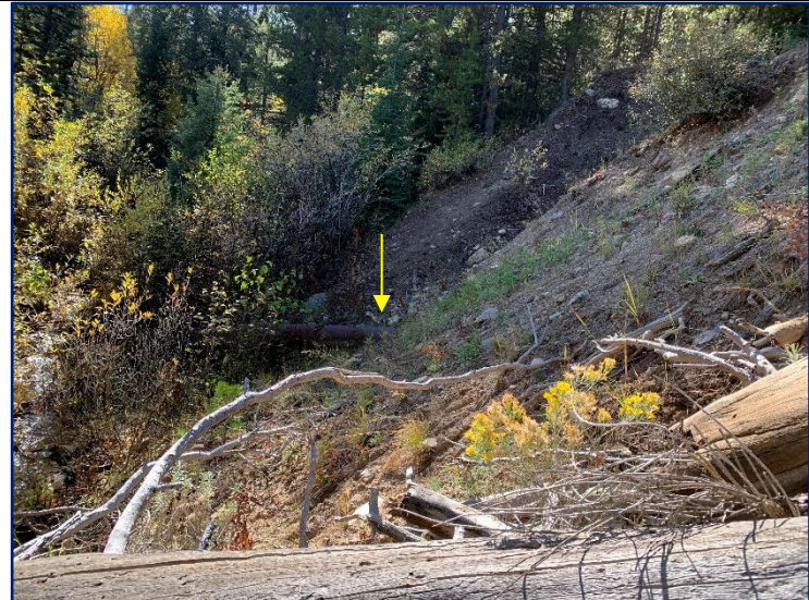
"Before" photo of first high and eroding bank. Looking south.
