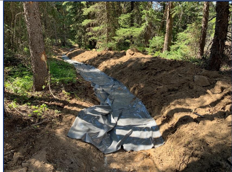
Installation of 30mi PVC plastic lining in temporary stream diversion.
