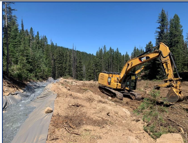
Subgrade excavation near the top of the project area.
