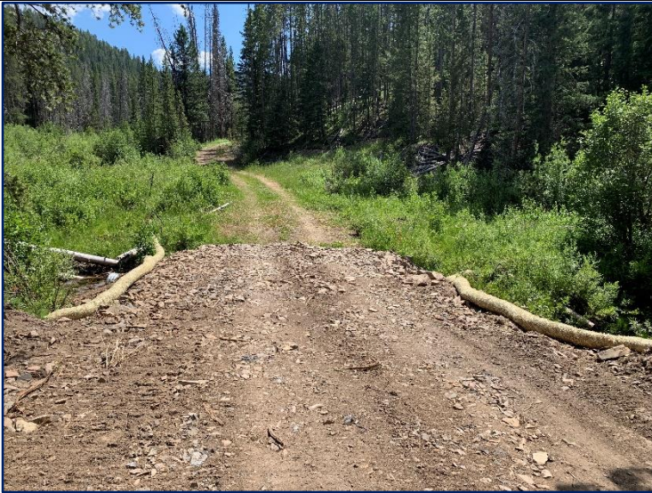
First stream crossing and straw wattle BMP entering the project area.
