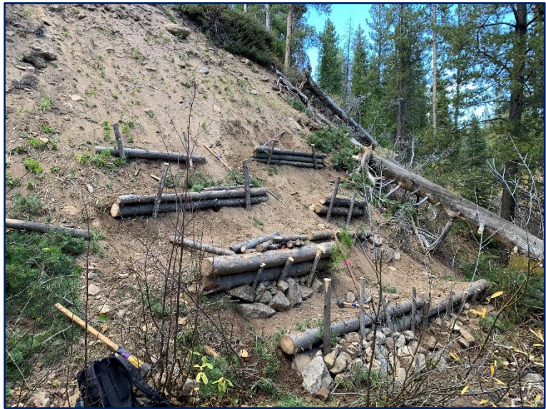
Mid stabilization/wattle fence construction.
