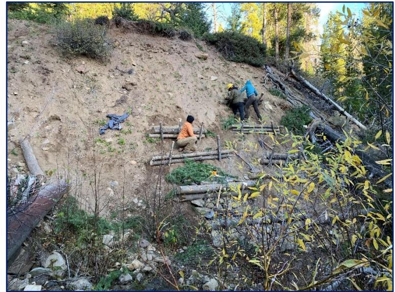
MCC crews working up high on the steep, eroding hillside/bank.
