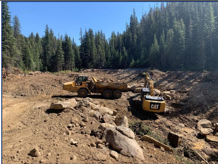
Excavator loading haul truck to be sent to the fill area.
