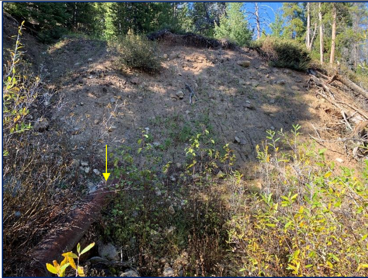
"Before" photo of the first high and eroding bank. Looking west.
