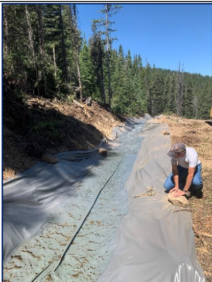
Temporary diversion soon after stream flow was activated.
