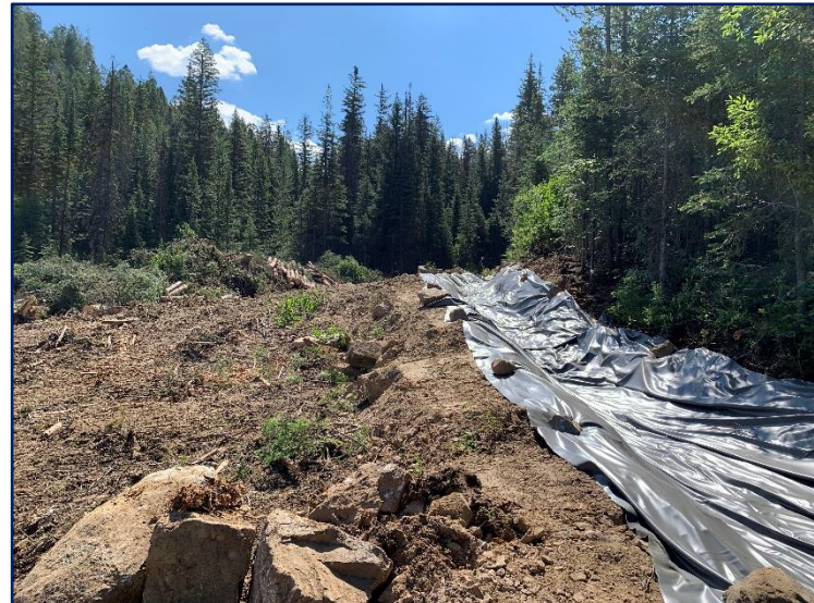
Temporary diversion ditch next to project site before activation
