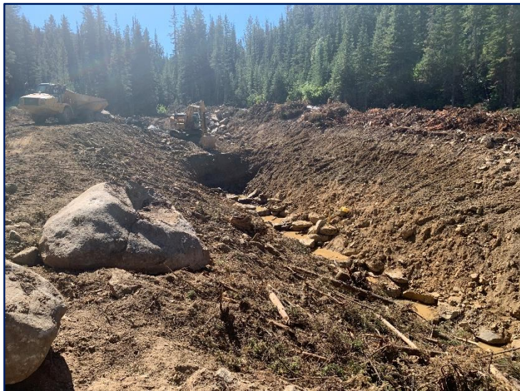
Roughly halfway through construction, before encountering the hard rock layer
