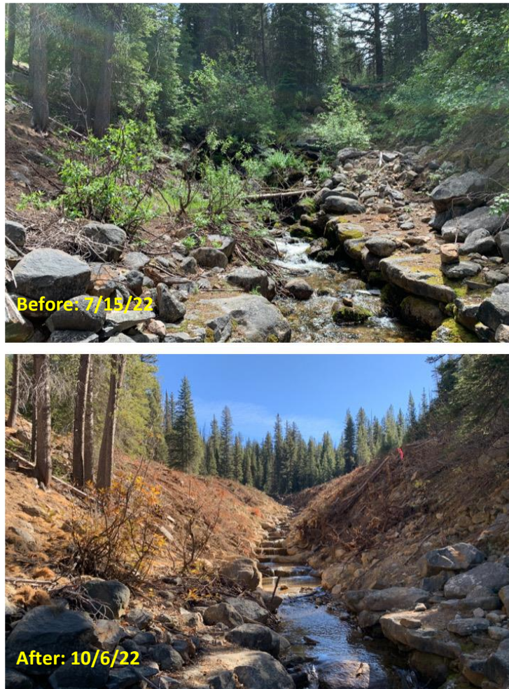
Figure 4. Before and after photo of the completed project, looking upstream.
