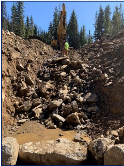
Bedrock layer broken up after the first use of the hydraulic jackhammer attachment.
