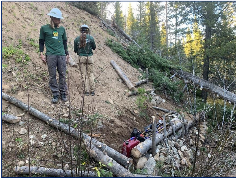
First wattle fence at the toe of the steep eroding bank.
