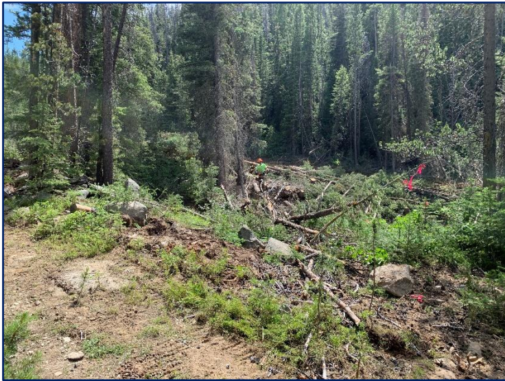
Clearing the project area of trees to enable room to work.
