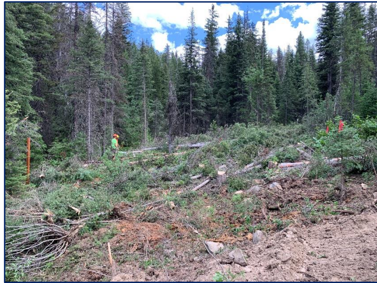
Cleared project area. Slashed was stockpiled for later use.
