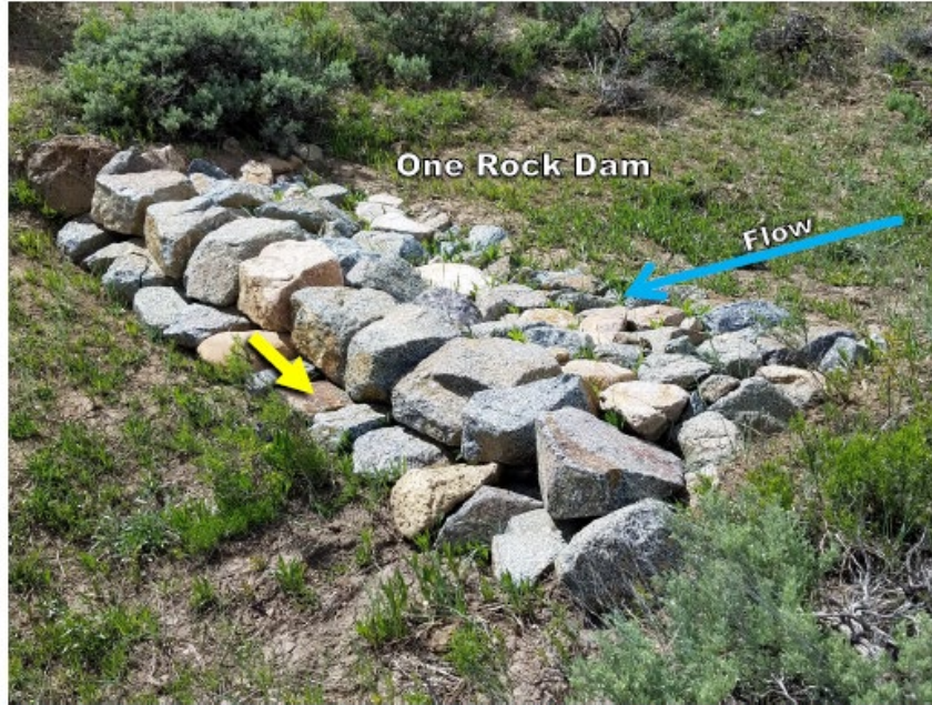
Figure 14. One rock dams should have a footer for splash apron on the downstream end that extends far enough to intercept water pouring over the structure in a high flow event (denoted by yellow arrow). Photo by: Nathan Seward
