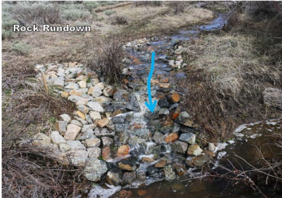
Figure 10. The center of a rock rundown should be the lowest so water runs down the middle and not around the structure. Photo by: Nathan Seward
