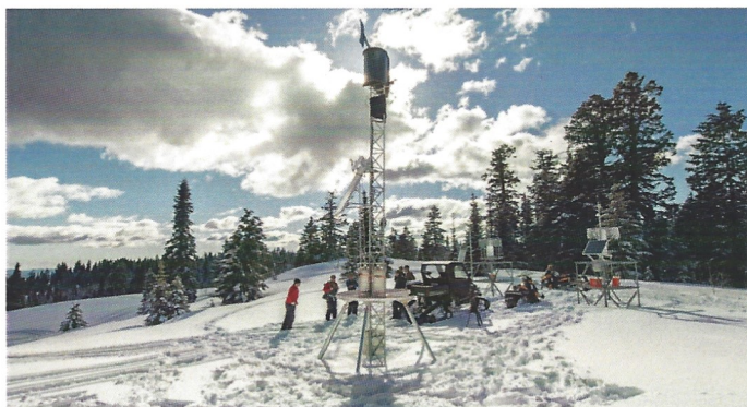
Ground-based generator Photo Courtesy Idaho Power Company
