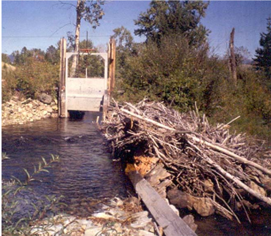
Company Ditch Headgate – Wise River flows from right to left.
