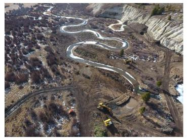
pacts, which left the old channel pinned against a high, eroding bank by a man-made dike feature. These human -caused alterations have caused 800+ tons of sediment per year to break away from the bank and fall into the stream, affecting downstream fish and mussel habitat. To fix the problem, we are constructing approximately 4,000 lineal feet of new stream channel east of the current channel through an area of healthy riparian vegetation.
