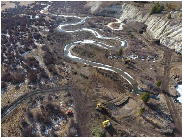
This is a much larger project, both in volume and length, than our previous stream restoration projects. Each meander, pool, riffle, bank, and floodplain are highly engineered to ensure a structurally stable stream, while also enhancing wildlife habitat. The project incorporated other water storage techniques as well, including depositional wetlands and floodplain micro-topography.
